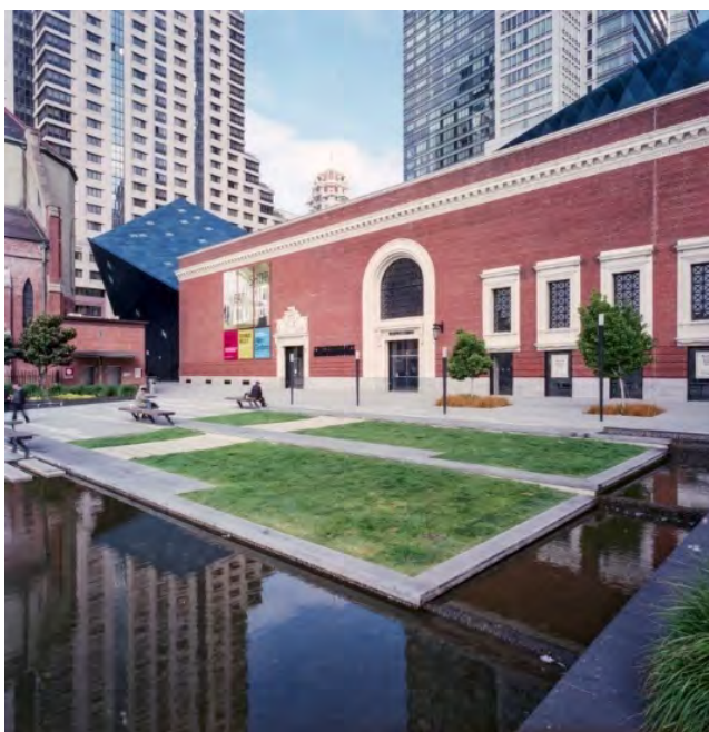
The Contemporary Jewish Museum fuses the 1907 Jessie Street Power Substation, designed by Willis Polk, with a projecting addition by Daniel Libeskind, completed in 2008 (credit: Jeremy Blakeslee)
